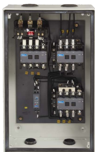
Interior View of MU FASD
