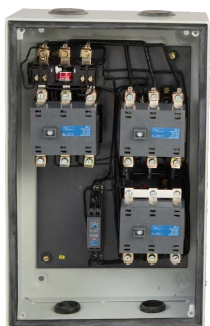
Interior View of ML FASD
